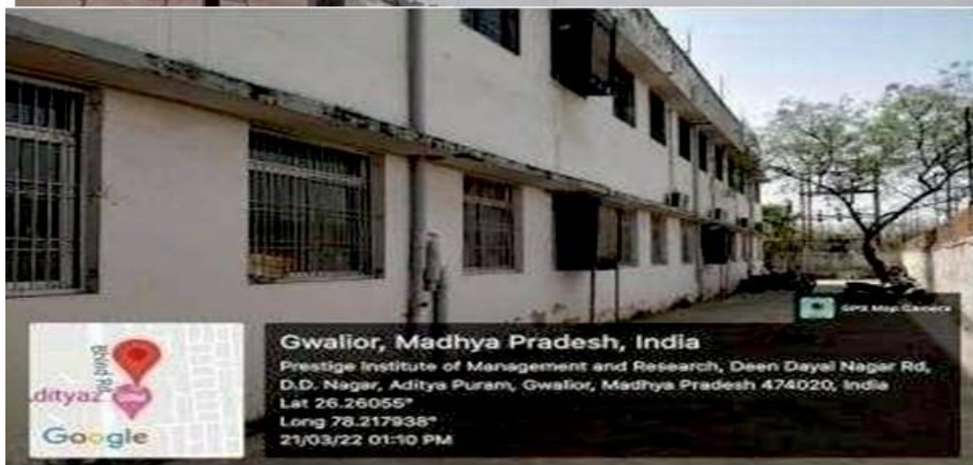
Waste Supply Pipe System in Block B
