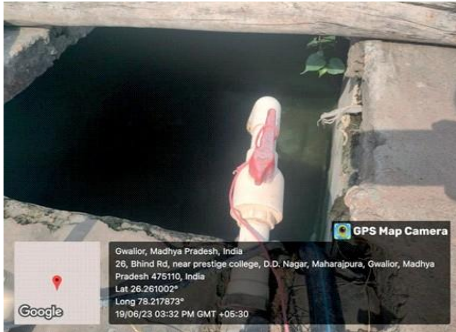
Underground Water tank in front of Block C Ground Area
