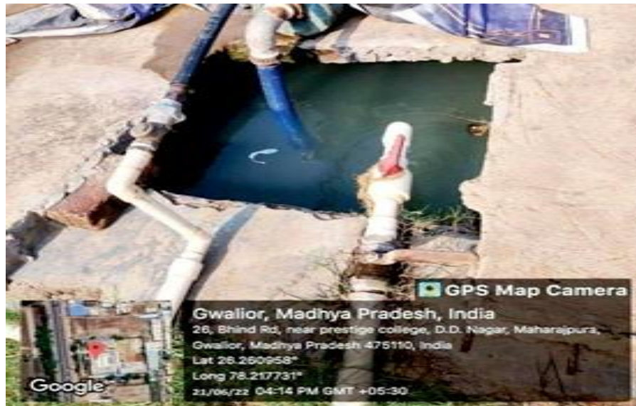
Underground Water tank in front of Block C Ground Area
